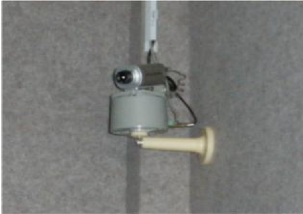
Camera CCTV Rotary di Ruang Praktikum
